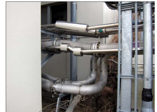
↑ Distortion of bellows
