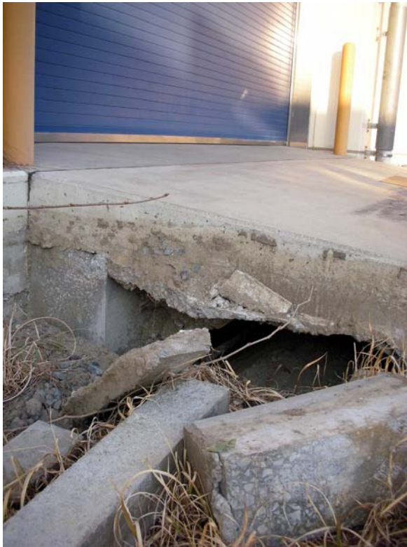
Entrance of the loading deck. Already repaired.
